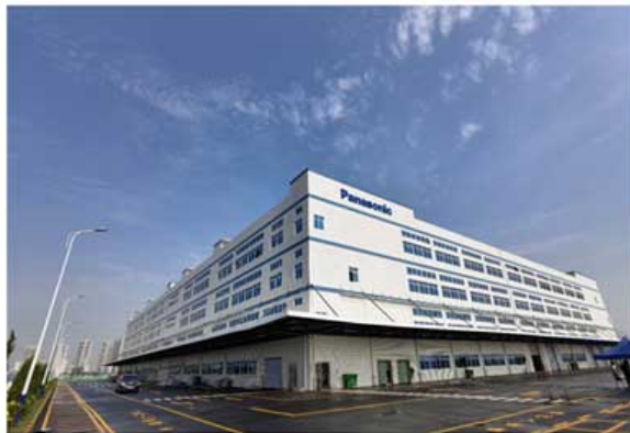
General view of the plant
